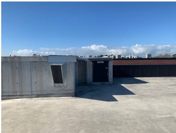
existing lift and stair overrun and half-height door to stair
