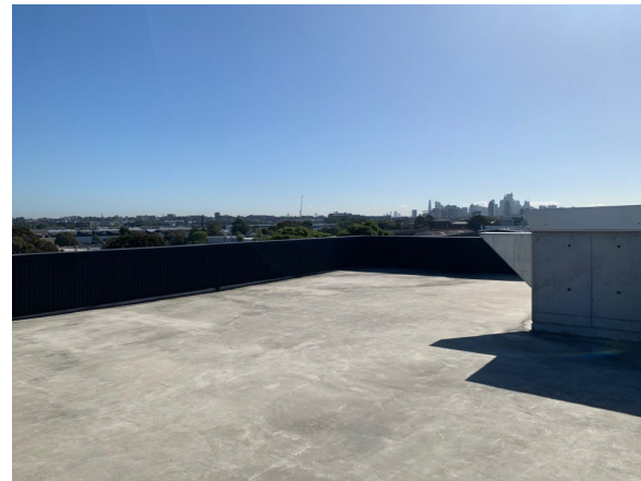
north-west corner of rooftop
