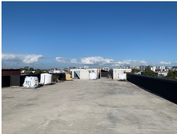
southern end of rooftop
